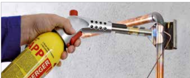
Brazing in gas installation
