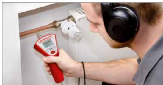
Acoustic leak detection of heating installations
