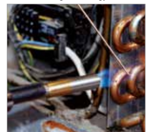
Brazing in refrigeration / air-conditioning technology
