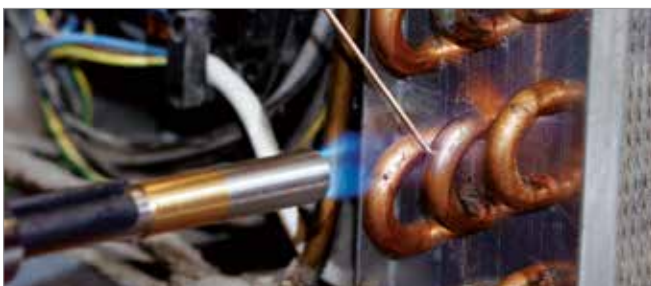
Brazing in refrigeration / air-conditioning technology
