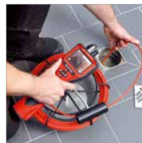
Inspection of floor drains
