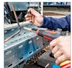
Brazing in refrigeration / air-conditioning technology
